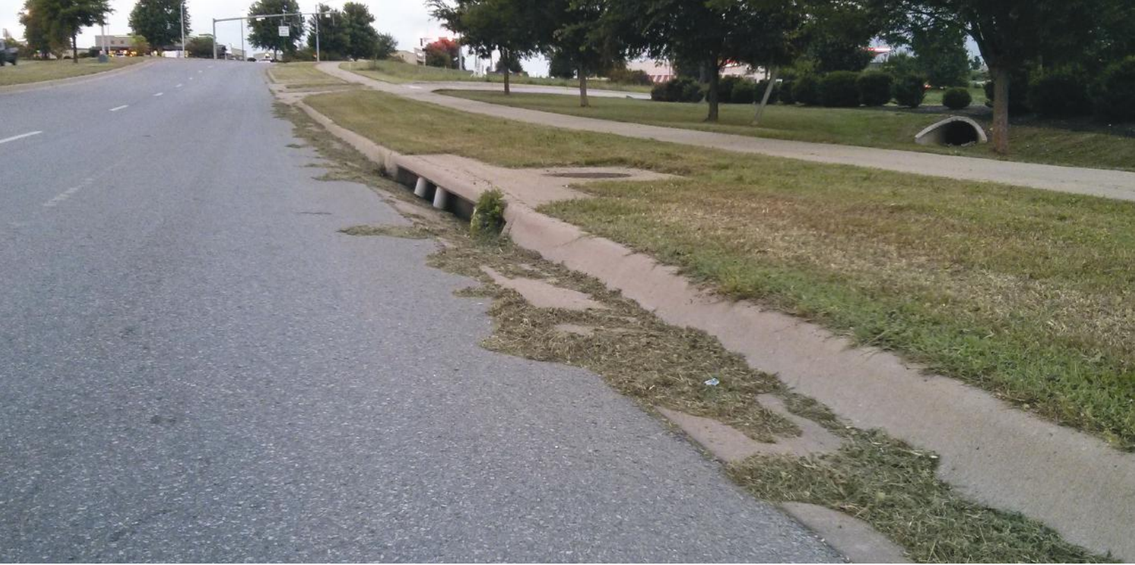
Image caption: Grass clippings on roads can be washed into the stormdrain when it rains, and can cause pollution in receiving streams.
